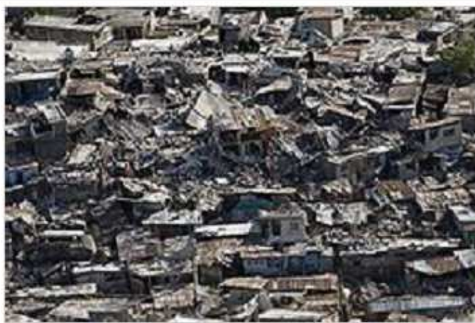
Damaged buildings in Port-au-Prince, Haiti, January 2010.
